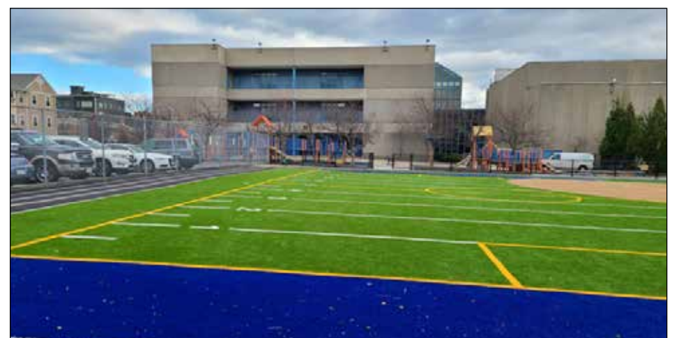
The Boston Parks and Recreation recently completed several field and playground renovation projects citywide including Orton Field at 200 D Street in South Boston. The fencing, synthetic turf, and entrances were all upgraded under Mayor Walsh's Capital Improvement Plan.
